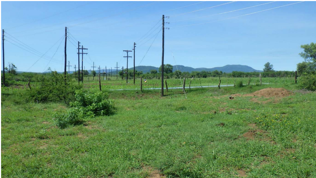
Figure 8: View of the corridor near the Spencer substation.
